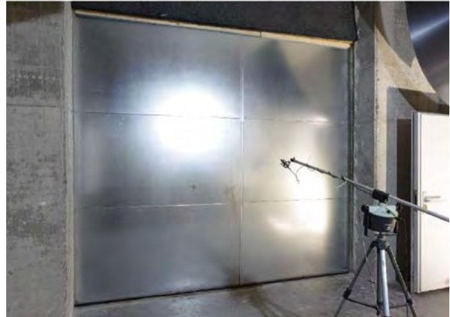
rear wall in the receiving room
